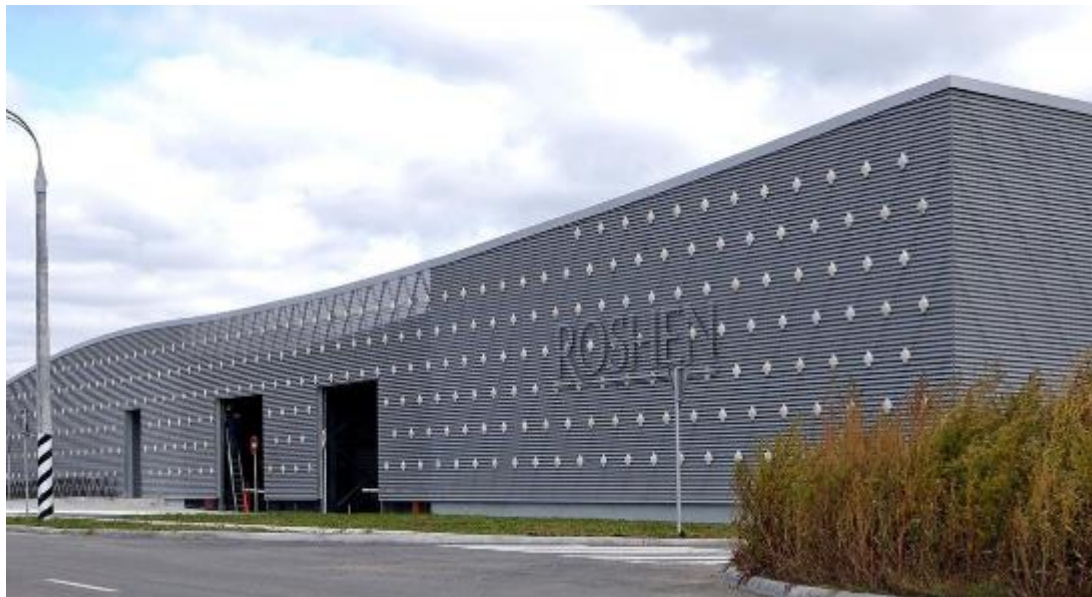
Figure 2.3 – PJSC Vinnytsia Dairy Plant Roshen
