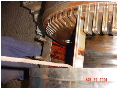
Fig. 1 Driven side view of flexible coupling with heavy damaged plates
